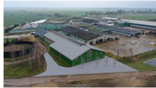
Dairy Farm modernization project
